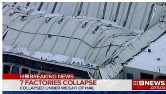
Figure 9 – Photographs of collapsed warehouses 25 April 2015, Sydney.
