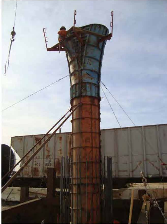
Figure 2.18: Column Forms with Temporary Support installed
