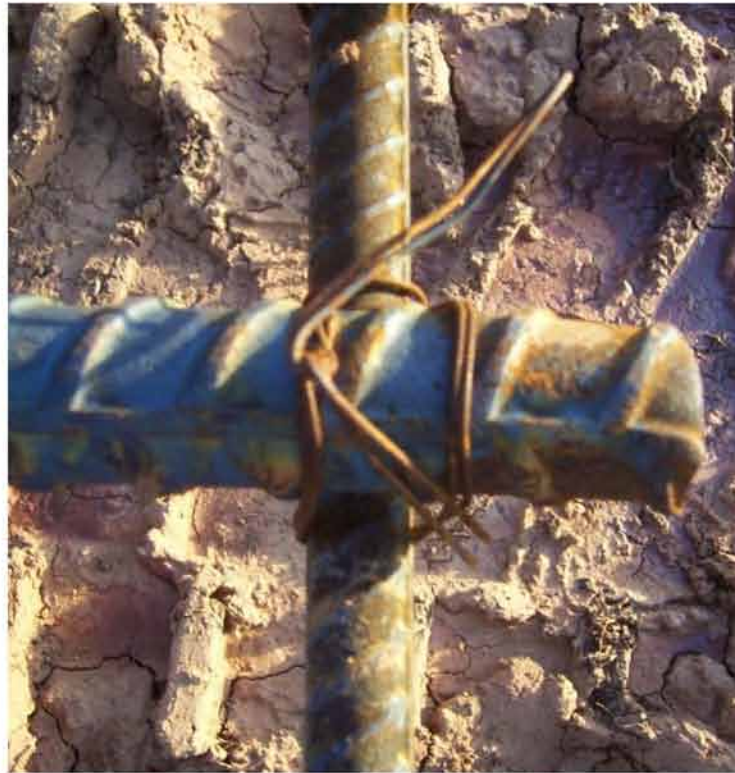
Figure 2.9: Double-U Tie Wire Connection
