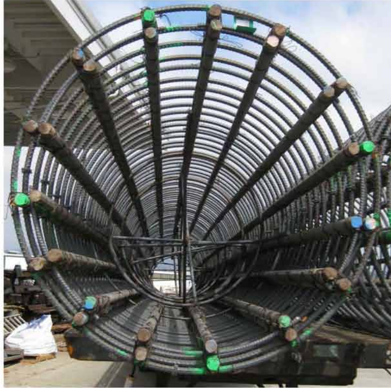
Figure 2.2: Pick-up Bars in a Column Rebar Cage
