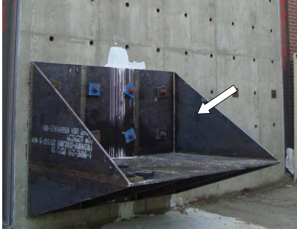
Figure 3.54: Details of Steel Bracket Attachment
