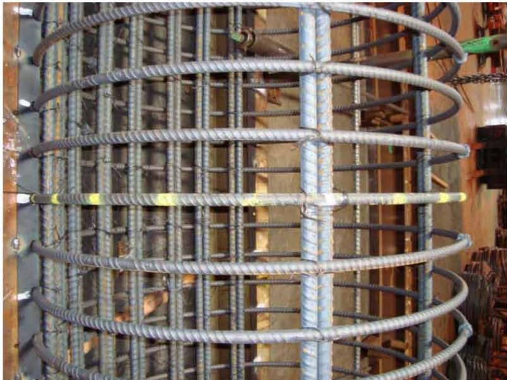
Figure 2.3: Template-hoops in a Column Rebar Cage
