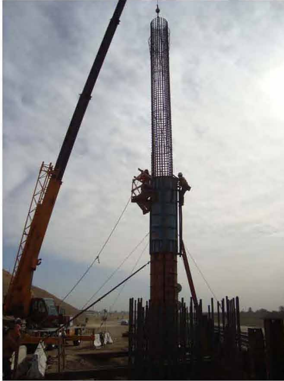
Figure 2.20: Column Rebar Cage being set inside the Column Forms
