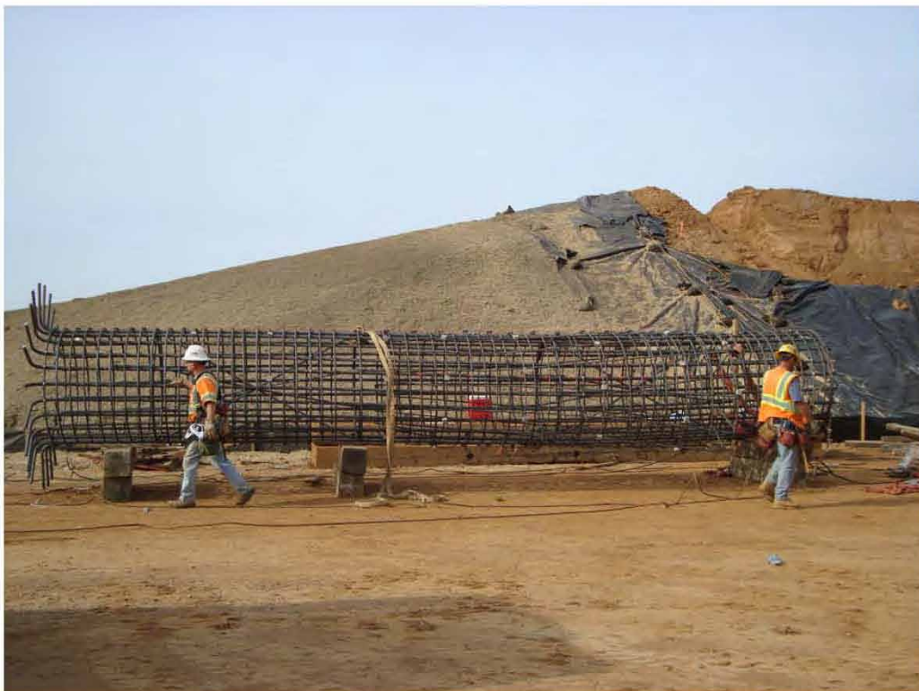
Figure 2.21: Rebar Cage with two X-braces ready to be lifted
