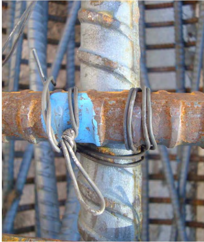
Figure 2.10: Wrap-and-Saddle Tie Wire Connection
