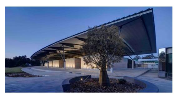
The main focus of the project is 6 distinctive rammed earth vaults, designed to be able to shield the botanical collection from bushfires and extreme temperatures.
