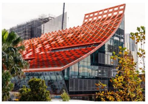
Northrop were engaged to complete the structural engineering design of the building which included an innovative triangular shape design sculpted to match the course of the winter sun. Northrop designed a bespoke structural steel roof frame to supports the envelope of the building, forming both the roof and façade made of hundreds of individual insulated roof panels.
