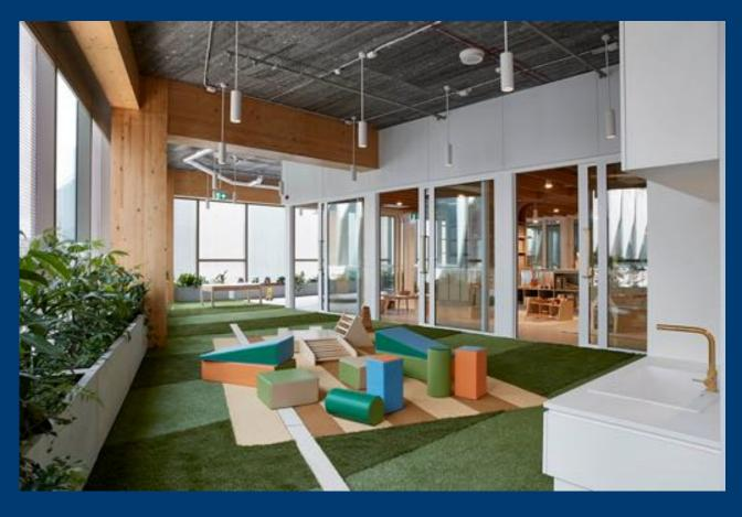
The building consists of a glulam beam and column structure with CLT slabs throughout. The extensive use of timber has dramatically reduced the embodied carbon footprint of the building structure, by saving an estimated 1200T of CO2 when compared to a conventional concrete building.
