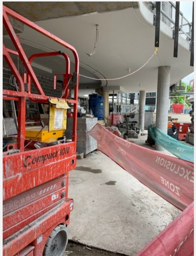
Photo 5: New walkway column locations adjusted to sit over existing structure
